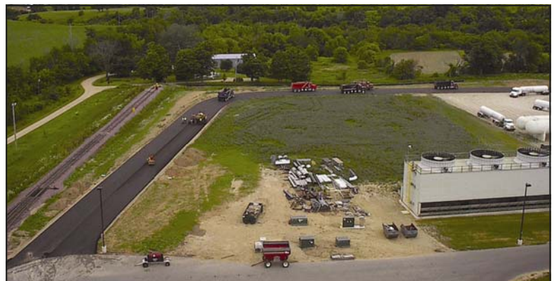
New staging road for corn and DDG trucks
